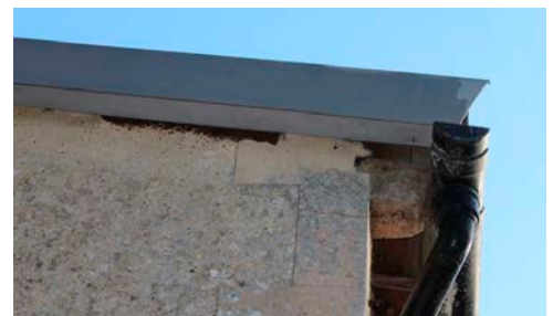
Figure 11: End of fascia with acute corner and incomplete closure
