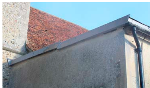
Figure 10: Straight verge fascia contrasts with uneven masonry
