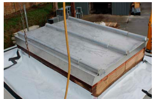
Figure 6: Round batten-roll roof sample under test
